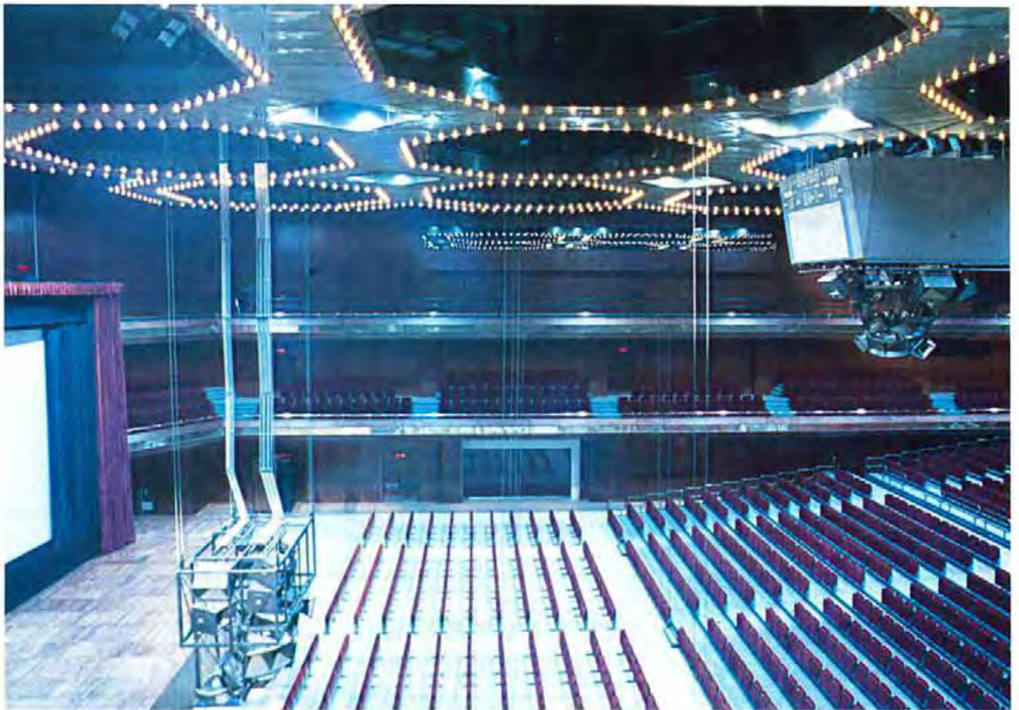
Main auditorium of the Putra Centre showing house lighting using "egg crate" system, retractable seating, sound cluster in front of stage (in lowered position), electronic scoreboard and sound cluster in centre of arena area, and projection screen.
